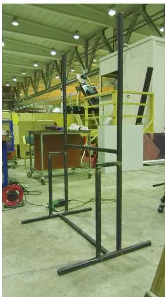
Figure 3.2: Steel frame for marshalling cabinet.
