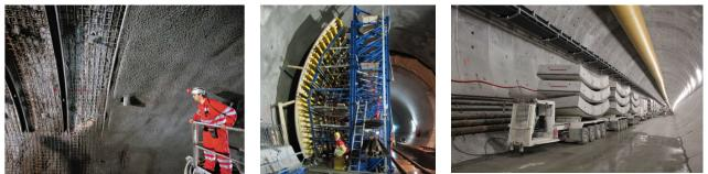
Figure 2-39: Three used tunnel lining methods. Left: Shotcrete (2-20 mm) reinforced[94]. Middle: CIP concrete lining [95]. Right: Concrete segments(30-50mm) [96]. A tunnel lining can also include both shotcrete and CIP.
