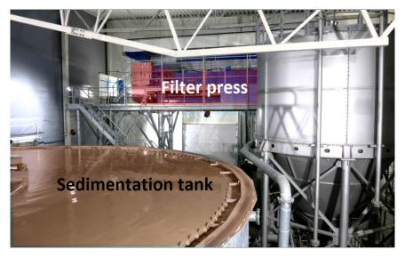
Figure 2-16: At the Follo line project(figure) and AlpTransit projects the cleansing of sludge from the wet processing of TBM spoil was done by a clarifier (sedimentation tank) and a VPA (filter press) creating filter cakes of mud for the landfill. The partially cleansed water can be used back in the wet processing.
