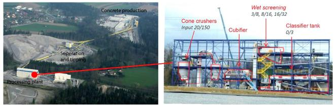
Figure 2-33: Left: Overview over Koralm KAT2. Showing the concrete production at tunnel portal. Secondly, separation and tipping of spoil (0/16 and 16/150). At last processing of spoil and storage. All connected by a conveyer system[22]. Right: The building of the processing plant and installing of the machinery.
