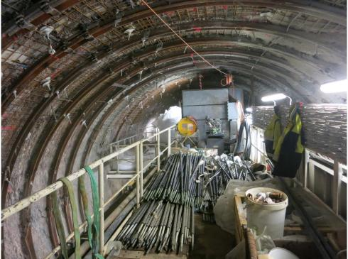
Figure 2-32: In a weakness zone. Securing the tunnel lining before shotcrete are applied in the new Ulriken tunnel
