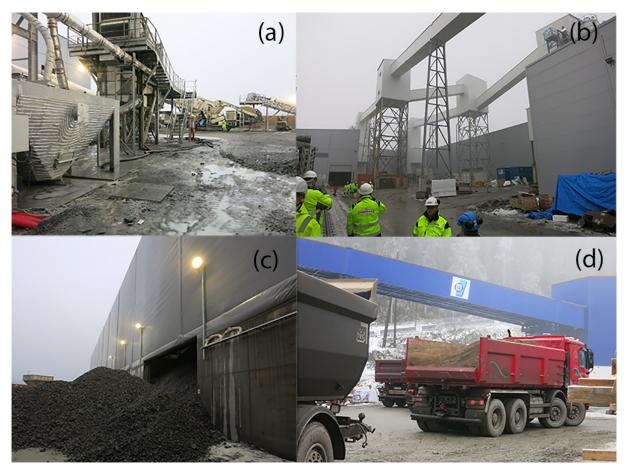
Figure 3-2: (a) Processing facility at the follo line project, dewatering cyclone can be seen in front, in the back a mobile screener combined with a cone crusher. (b) Conveyer system, concrete batching plants and segment production. (c) High quality spoil, this would be transported by wheel loader into the scalping screen and material processing. (d) Constant delivery of third party aggregates for concrete production.
