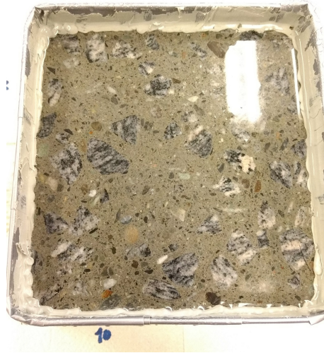
Figure E83: Damages, Sample 10, Series 2
