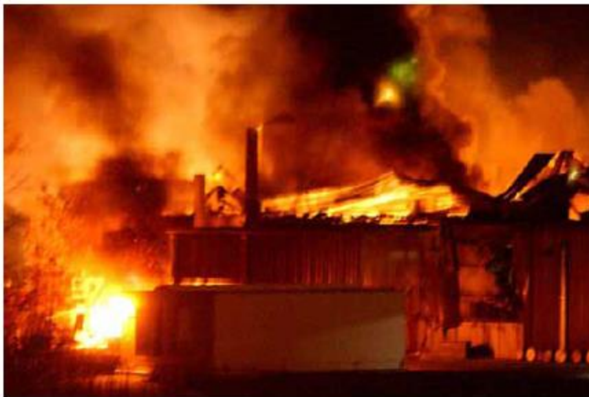
Figure 13: Intense fire following an aluminium dust explosion at Hayes Lemmerz International (Huntington, Indiana, October 29, 2003).
