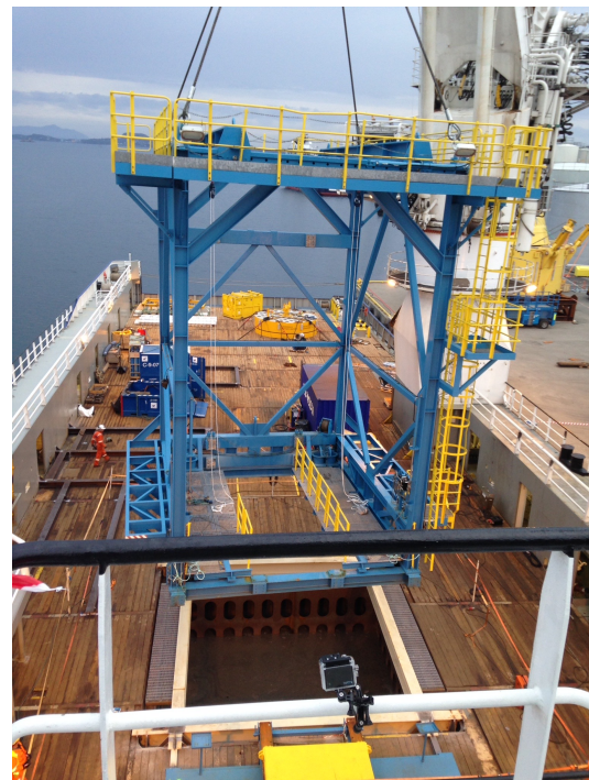
Figure 3.4: Tower installation over moonpool
