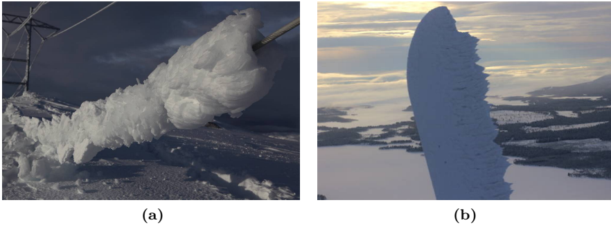
Figure 1.1: Examples of icing on outdoor infrastructure. (a) shows the grounded wire of an overhead transmission line that has broken down due to a large ice load[13]. (b) shows ice build up on a wind turbine blade[14].
