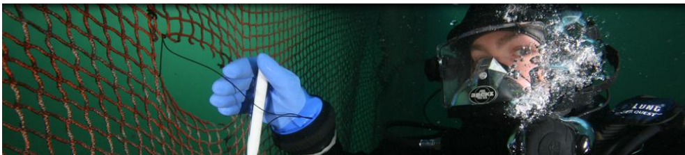
Figure 2.3: Repair of holes by a diver (internet).
