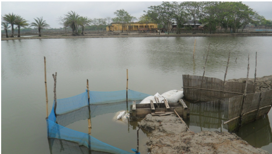
Fig 2: A sluice gate (indigenous technology) for taking in brackish water to a shrimp farm.
