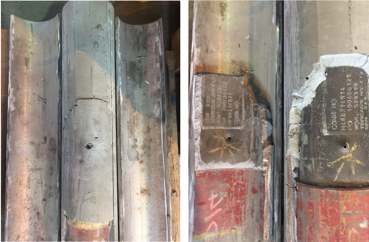
(a) Showing perforation through the cement.
