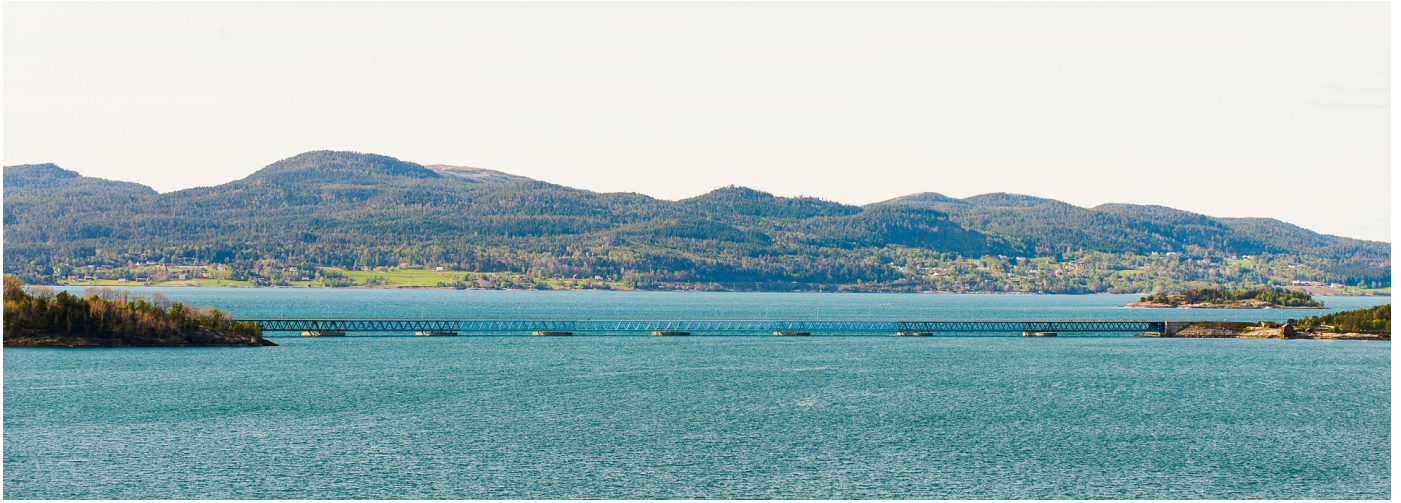
Figure 2: The Bergsøysund Bridge. Photograph by NTNU/K.A. Kvåle.
