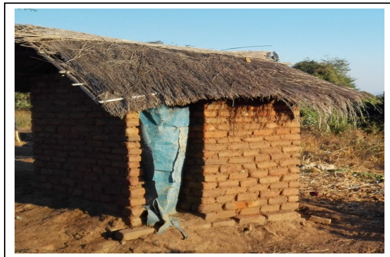
Figure 6.3 Pit latrine in Sadzi (Source: Fieldwork, Zomba 2015)
