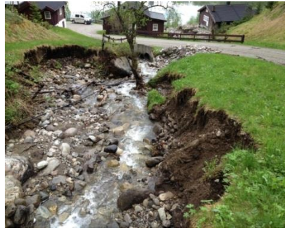
Figure 30: Damage point 4 (Foto: JBV v/Steinar Myrabø)
