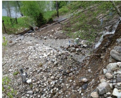
Figure 33: Damage point 7 (Foto: JBV v/Steinar Myrabø)
