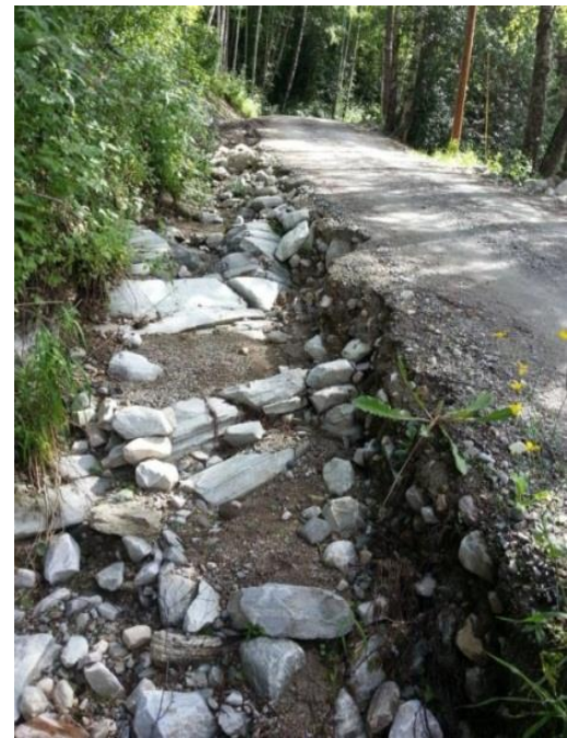
Figure 21: Probably due to a closed culvert in damage point 7 the water has followed the road and caused damages due to erosion (Photo: Steinar Myrabø)
