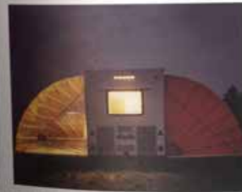
"The (Richard Buckminster Fuller) 'Newfound Wing', 1962-63, compact with fold-out rooms, with the sleeping area on the left and the living area on the right."
