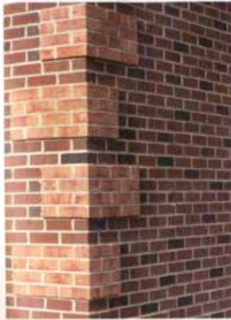
Figure 6-28 The brickwork at the corner projects to form brick quoins.
