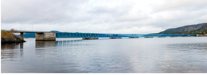
Figure 1: The Bergsøysund Bridge. Photograph: K. A. Kvåle.
