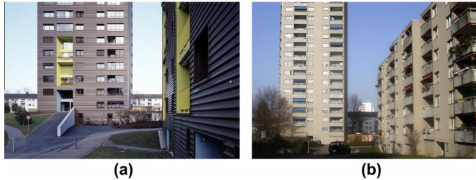
Figure 18. Changes in materialisation of facades and windows’ size and composition. Residential blocks, Zürich, Switzerland. Residential block after renovation (a). © [Andrea Helbling, Arazebra]. Reproduced by permission of Andrea Helbling, Arazebra, Zürich. Residential block before renovation (b). © [Schneider Studer Primas GmbH]. Reproduced by permission of Schneider Studer Primas GmbH.
