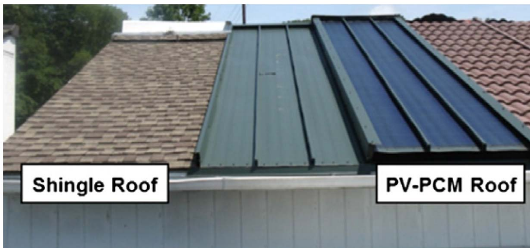
Figure 10 PV-PCM roof (Kosny et al. [62]).
