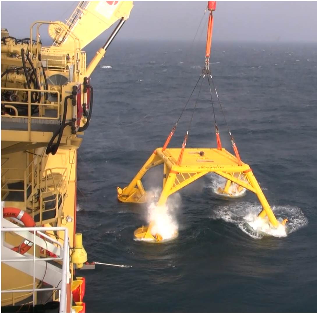
Figure 4.2: Installation of Fishing Protection Structure, courtesy of Storvik (2012)
