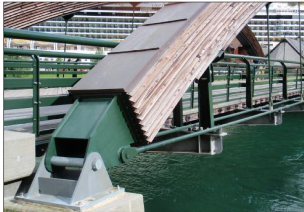
Figure 4.15 Structural weather protection on the arch [24]
