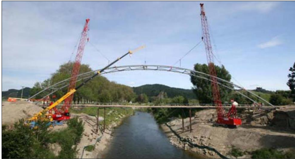
Figure 8.4 Erection of the arches with mobile cranes [47]
