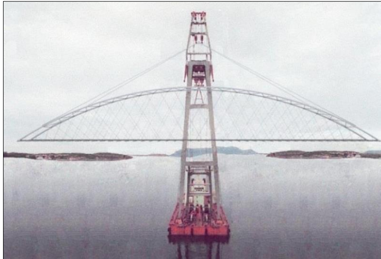
Figure 8.2 Åkvik Sound Bridge lifted in place by a floating crane [47]
