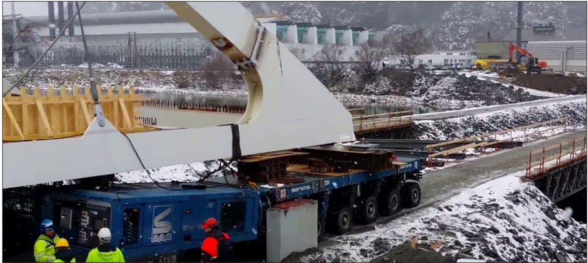
Figure 8.1 Transport of Driva Bridge [46]
