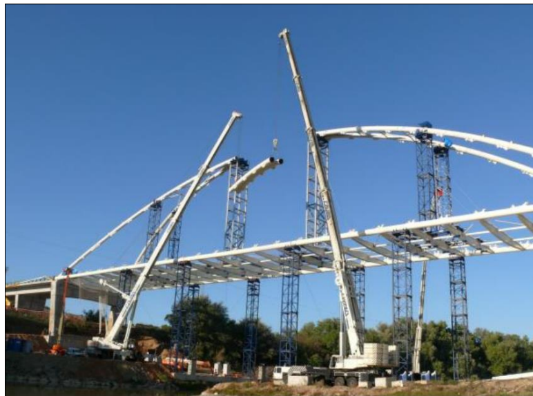
Figure 8.5 Erection of the arches with mobile cranes on temporary fillings [47]
