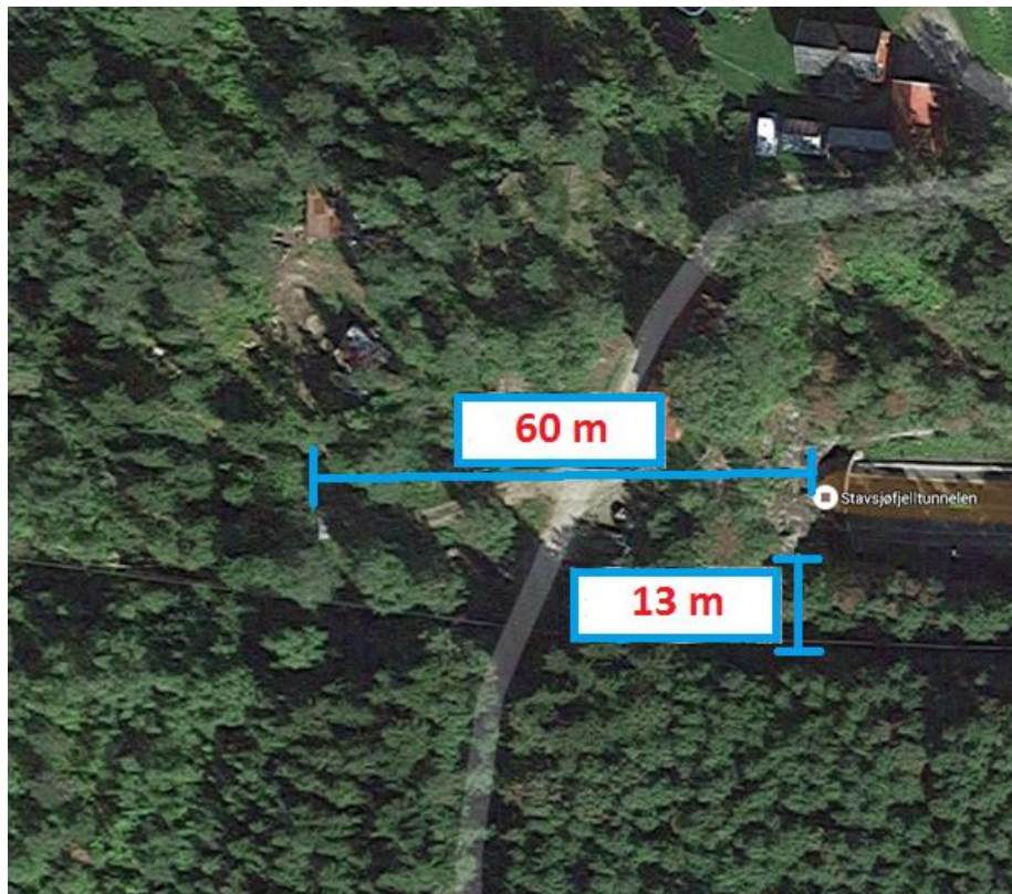
Figure 30 Aerial photo of the tunnel portal, direction Stjørdal
