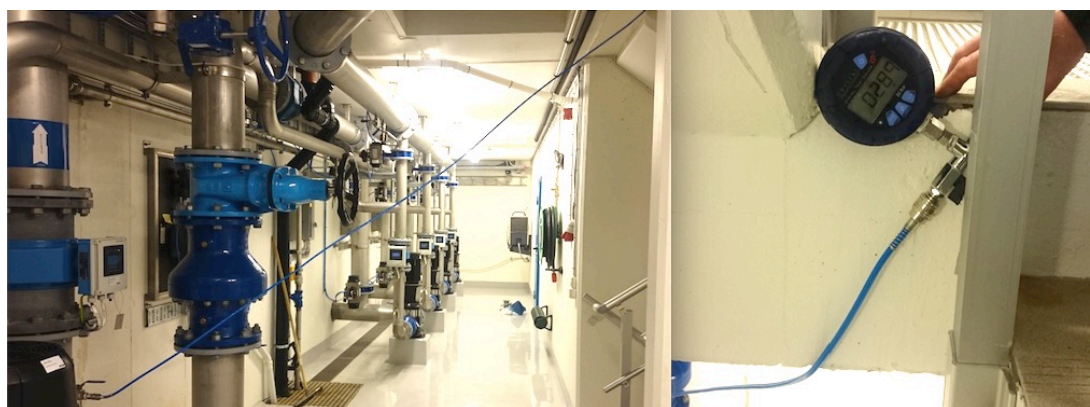
Figure 3.2.9: Difficult situation for reading pressure for pre/post static mixer.
