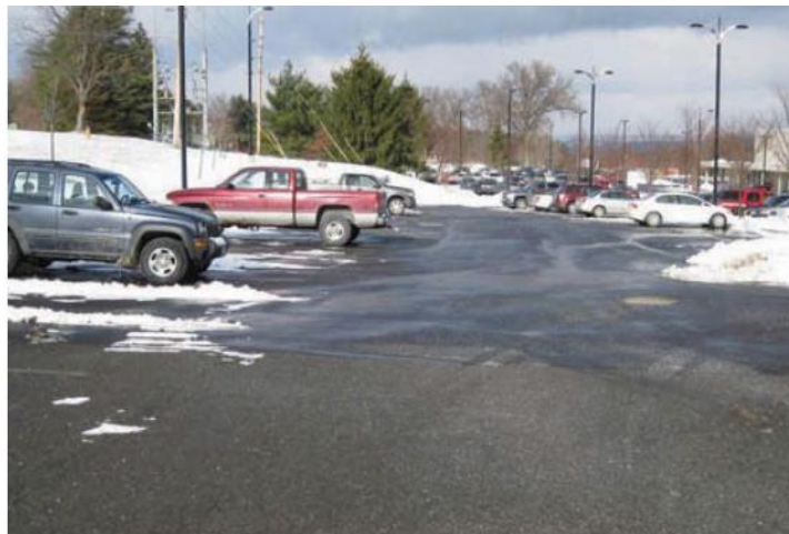
Figure 4 Dry porous asphalt close to the camera and regular asphalt further away from the camera (Eisenberg et al.) p. 55
