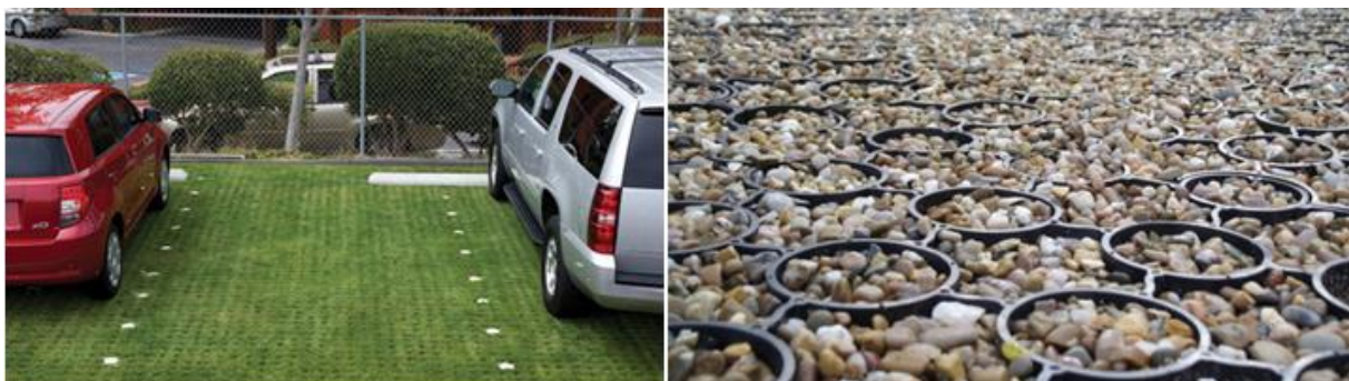
Figure 5 Grid pavement with grass to the left from (Dye, 2014) and aggregate to the right from (Ltd, 2015)
