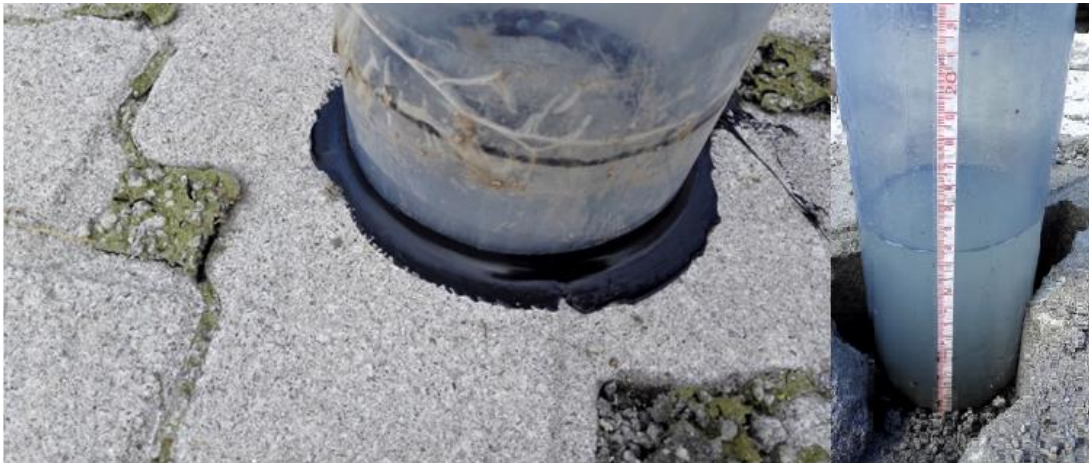
Figure 66 Left: picture of the sealing. Right: picture of the MPD placed in the bedding layer. (Photo: Jens H. Trandem)
