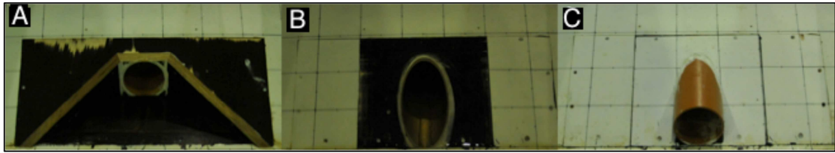
Figure 3.2 Culvert inlet shapes: A) Wingwalls, B) Cut inlet, C) Projecting inlet (Gotvassli, 2013)
