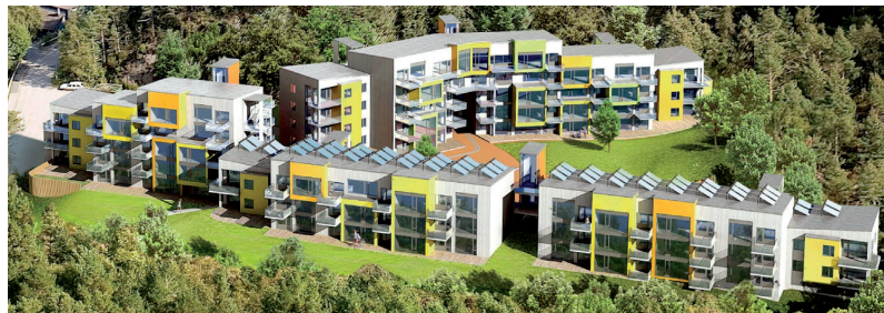
Fig. 1. Illustration of the Løvåshagen cooperative [26], showing low-energy apartments in the blocks to the left and back and passive house apartments in the two blocks in the front with solar thermal collectors on the roof.
