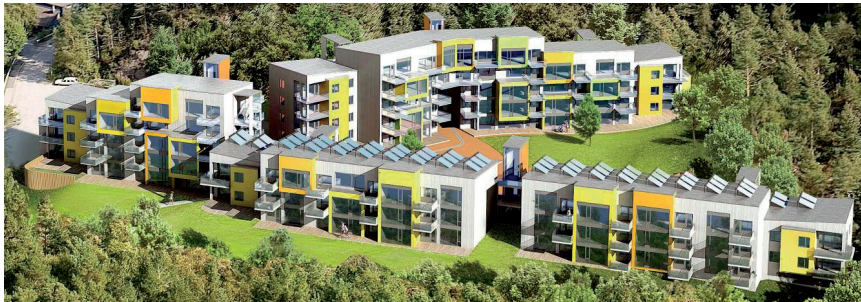
Figure 1 Illustration of Løvåshagen cooperative [ByBo AS 2009], showing low-energy apartments in the blocks to the left and back and passive house apartments in the two blocks in front with solar thermal collectors on the roof.
