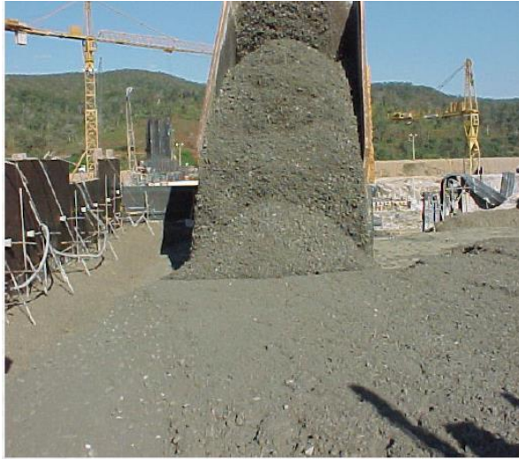
Figure 32 Unloading concrete by dump truck (Monteiro et .al)
