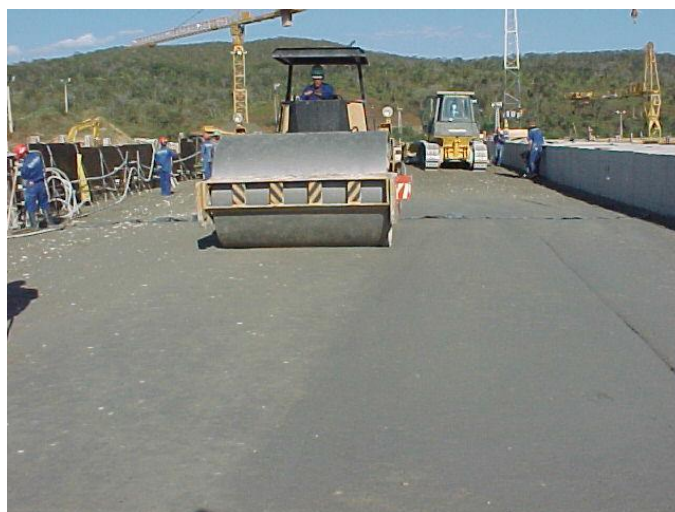
Figure 33 Spreading concrete by bulldozer (Monteiro et .al)
