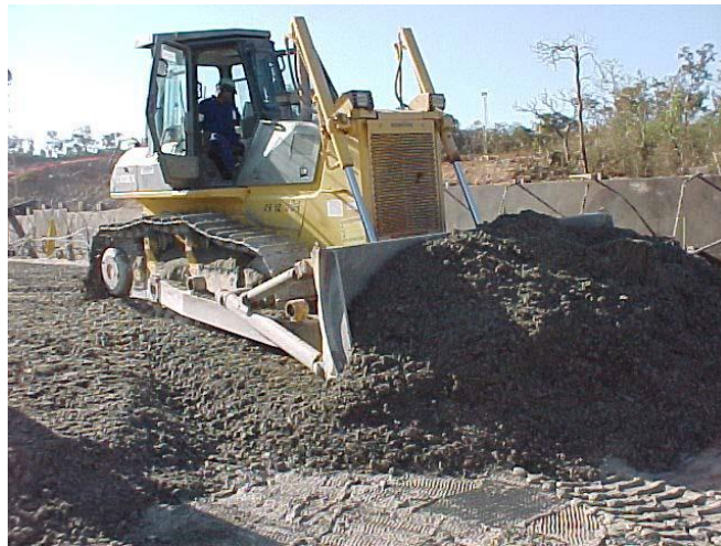
Figure 33 Spreading concrete by bulldozer (Monteiro et .al)
