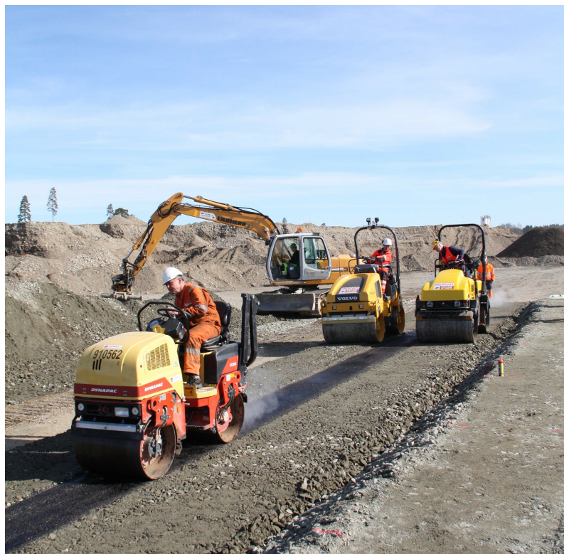
Figure 4.12: Simultaneous compaction of core and filters
