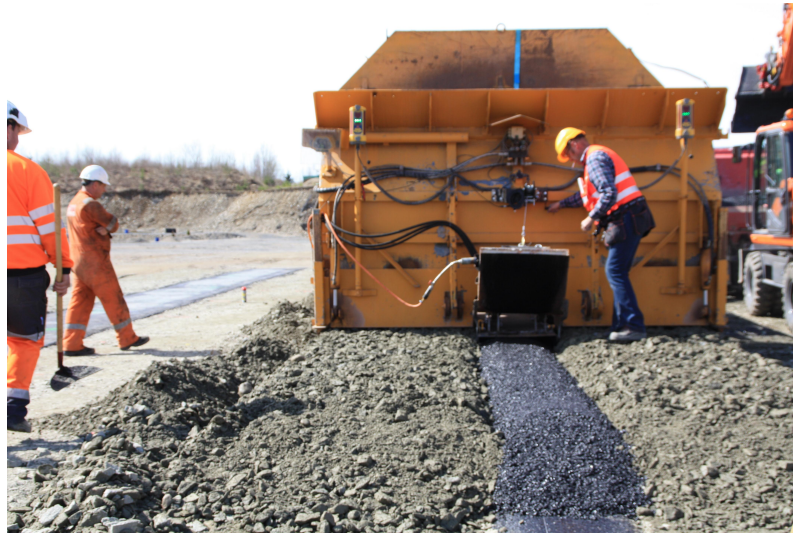
Figure 4.11: Placement of three layers simultaneously
