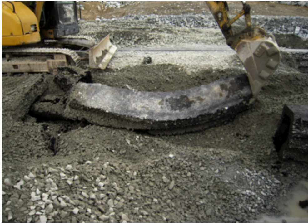
Figure 4.5: Ductility testing of the asphaltic core
