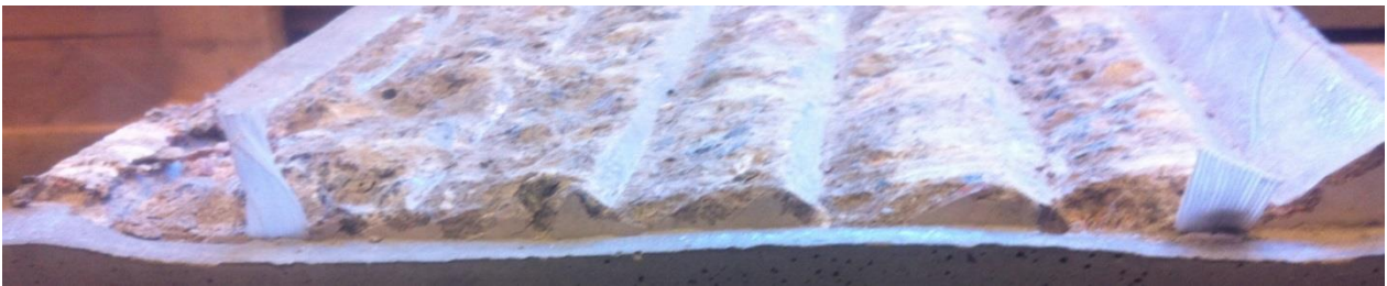
Figure 116. Test 1.3 Concrete asperities profile after the test.
