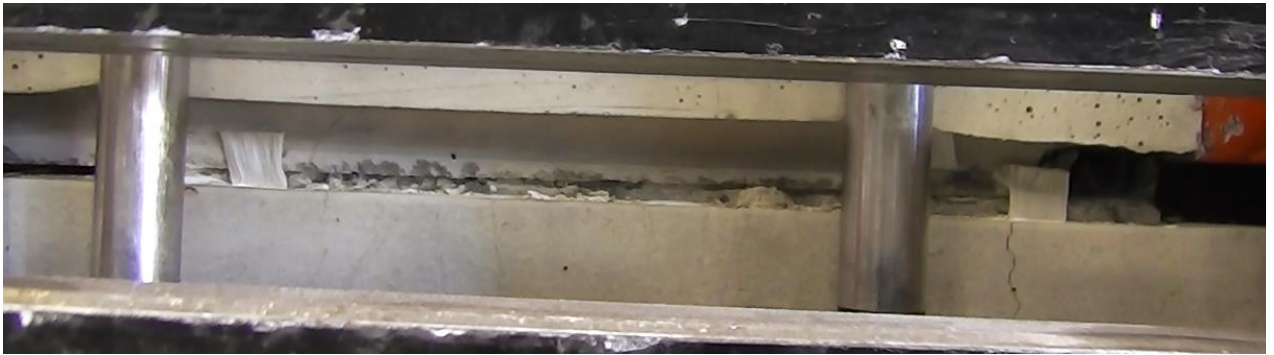
Figure 161. Test 4.2 after the test is finished.
