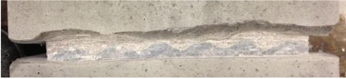
Figure 127. Test 2.1 before the test.
