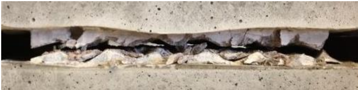
Figure 132. Test 2.2 after the test.
