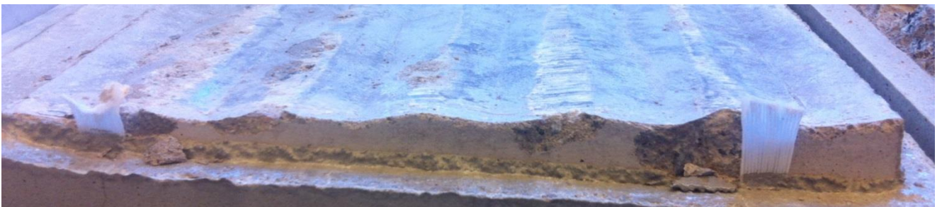
Figure 152. Test 3.3 Concrete asperities profile after the test.
