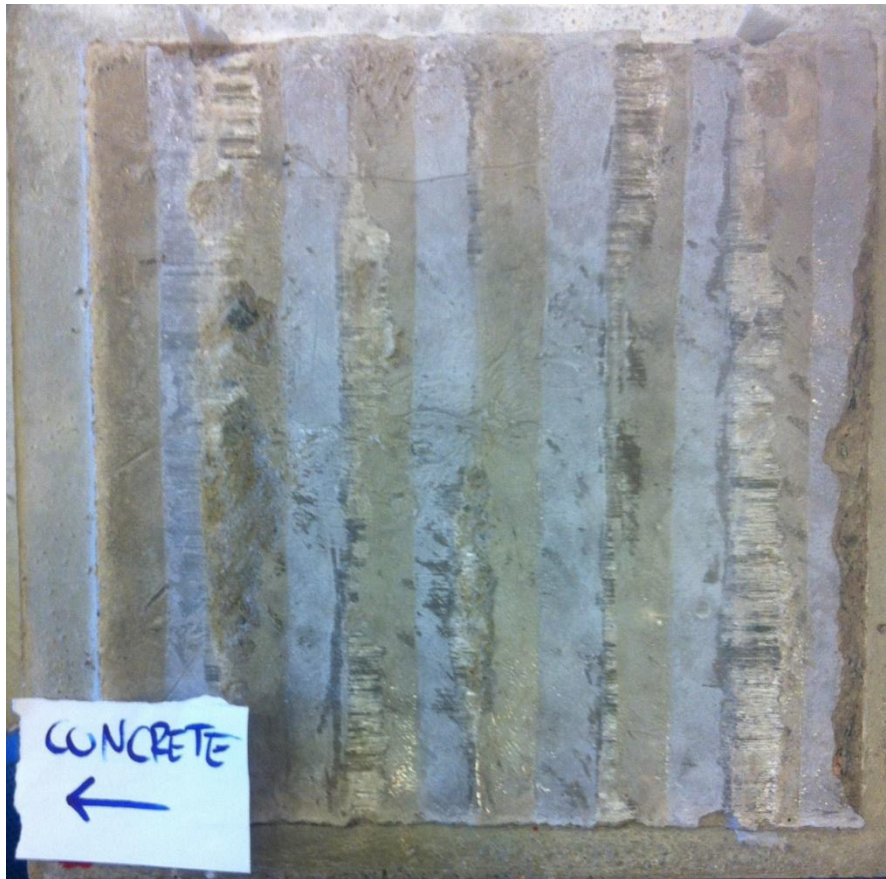
Figure 141. Test 3.2 Concrete interface after the test is finished.
