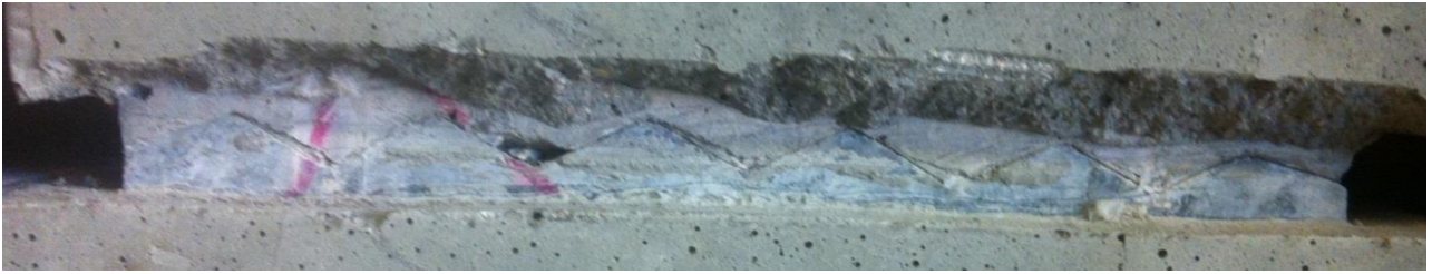
Figure 138. Test 2.3 before the test.
