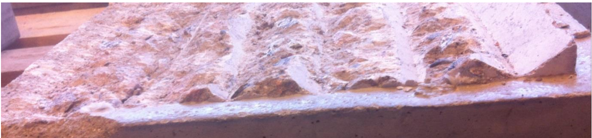
Figure 105. Test 1.1 Concrete asperities profile after the test.
