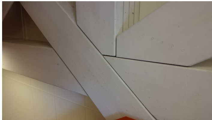
Figure 2.1: Glulam Connection
