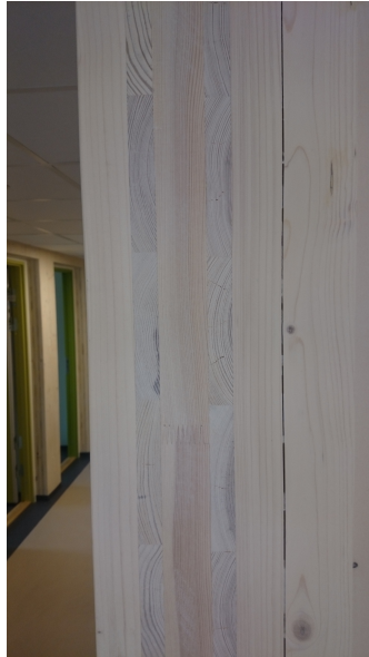
Figure 2.2: Cross laminated timber
