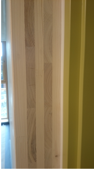
Figure 5.2: 120mm CLT at Moholt 50|50
