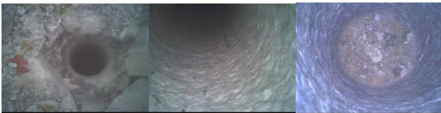
Figure 37 : clean performing of hammer drilling
