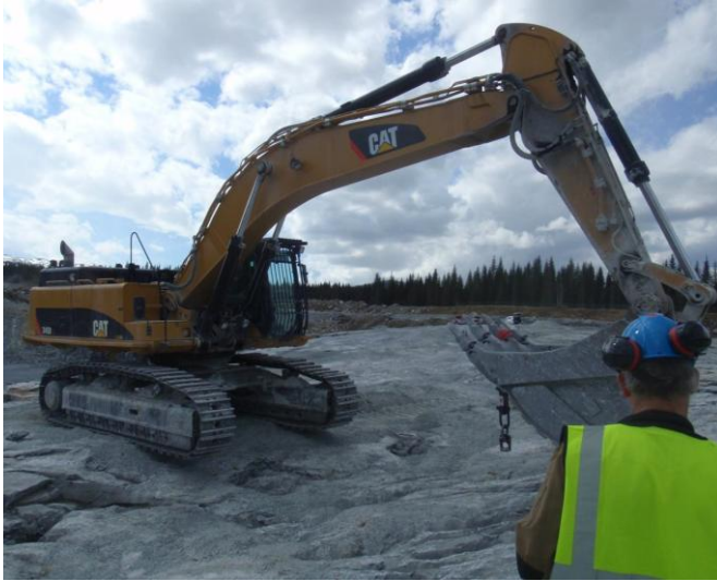
Figure 34 : Excavator CAT 450, Verdalskalk
