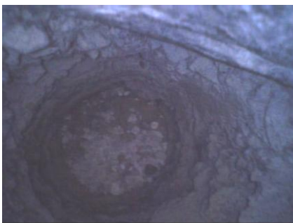
Figure 38 : 0,1 m long crushed rock zone under the fair rock surface at the bottom of the bolt nr13
