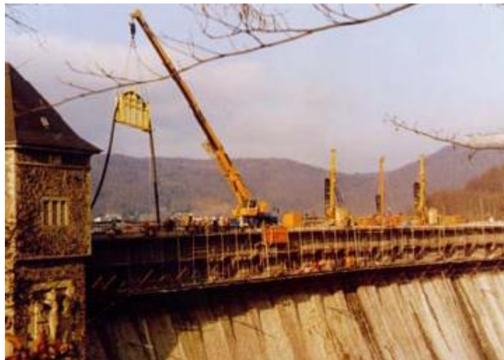
Figure 21 : Installation of anchor, Eder dam, after [1]
