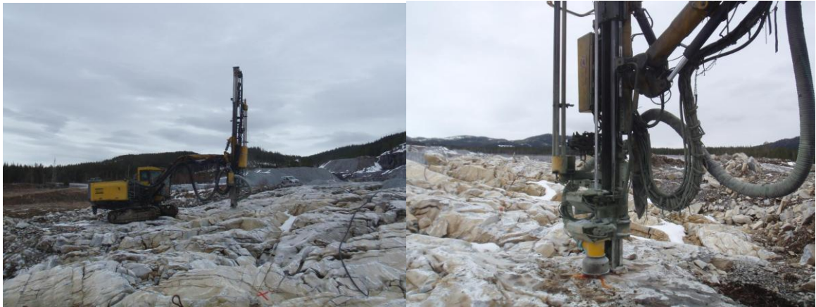
Figure 32 : Hammer drilling
