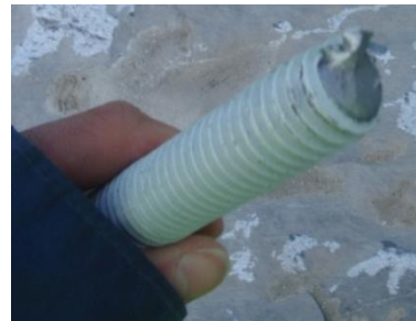
Break of the steel at the head of the bolt for loading higher than 23 tons
