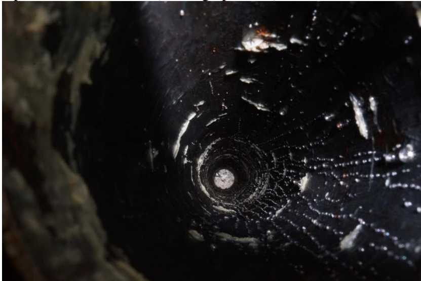
Pipe after wax removal (looking upstream):
