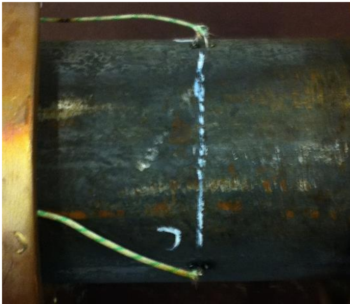
Figure H-1 - Type-K thermocouples welded to pipe surface
