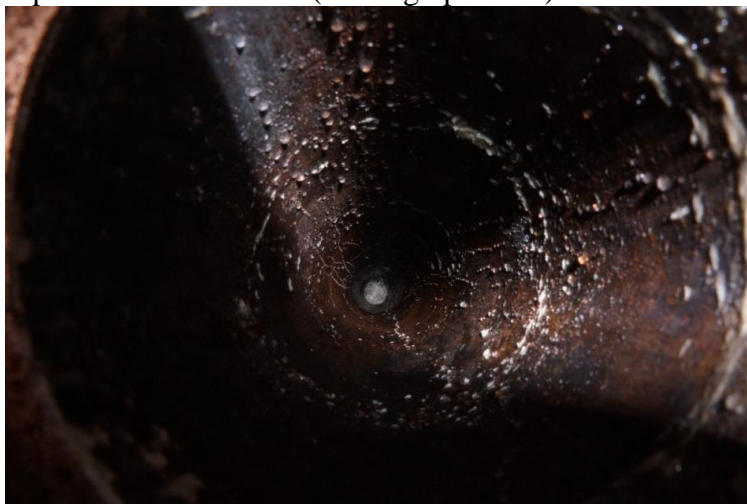
Pipe after wax removal (looking upstream):
