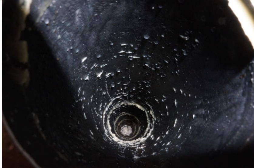
Pipe after wax removal (looking upstream):
