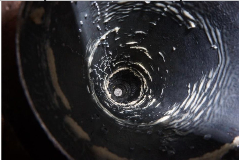
Figure 4-54 - Pipe after wax removal (looking downstream). Test 8: Pulse heating, 6 kW
