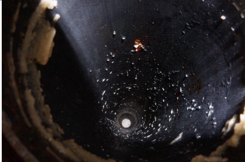
Pipe after wax removal (looking upstream):
