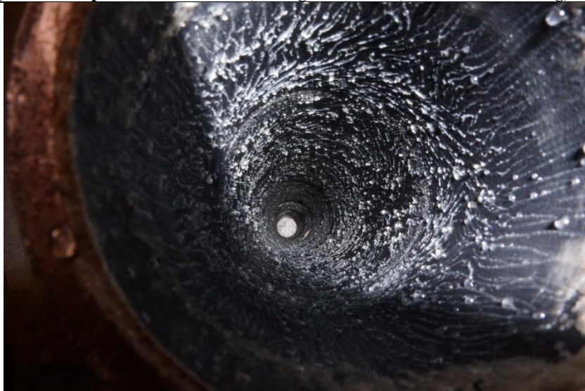
Figure 4-55 - Pipe after wax removal (looking upstream). Test 8: Pulse heating, 6 kW
