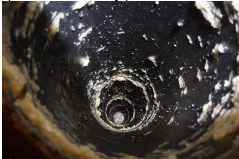
Pipe after wax removal (looking upstream):
