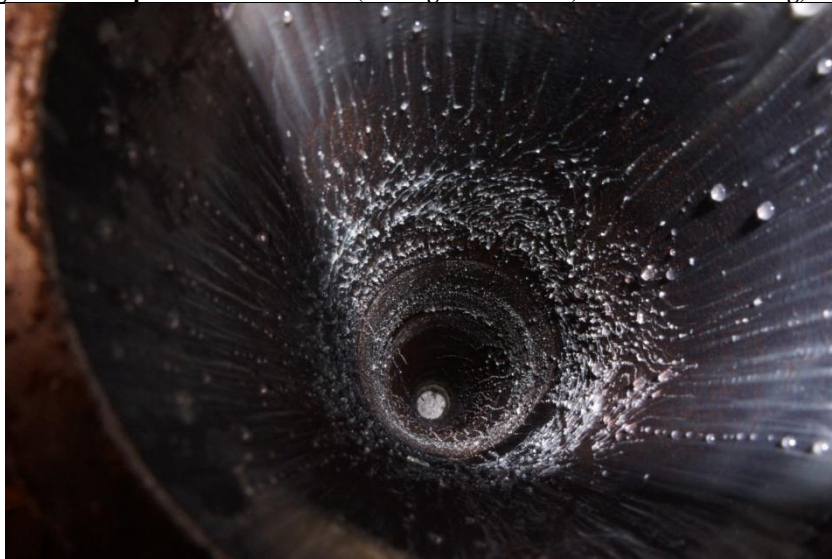
Figure 4-52 - Pipe after wax removal (looking upstream). Test 5: Scan heating, 6 kW
