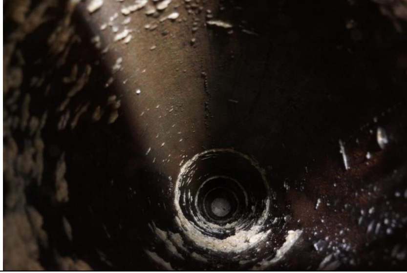
Pipe after wax removal (looking upstream):
