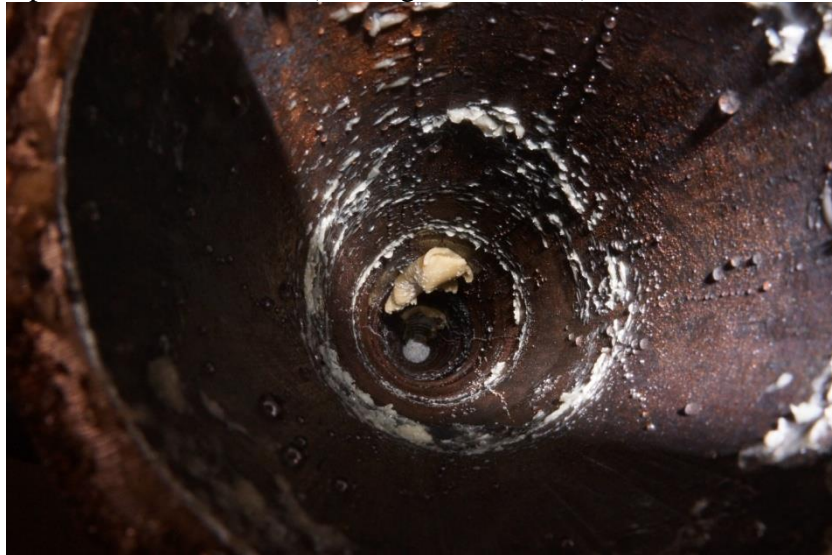
Pipe after wax removal (looking upstream):
