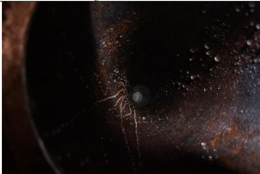
Figure 4-65 - Pipe after wax removal (looking downstream)
