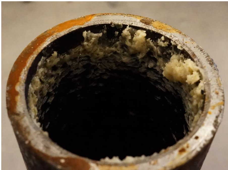
Figure 4-49 - Wax remains after wax removal. Looking upstream. Test 1.1: Upstream coil movement, 10 kW output power.
