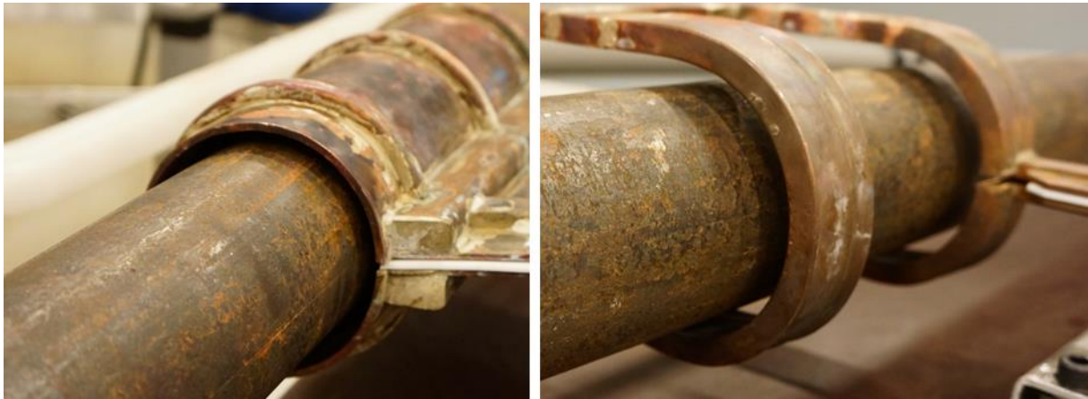
Figure 4-22 - Induction coil positioned over pipe
