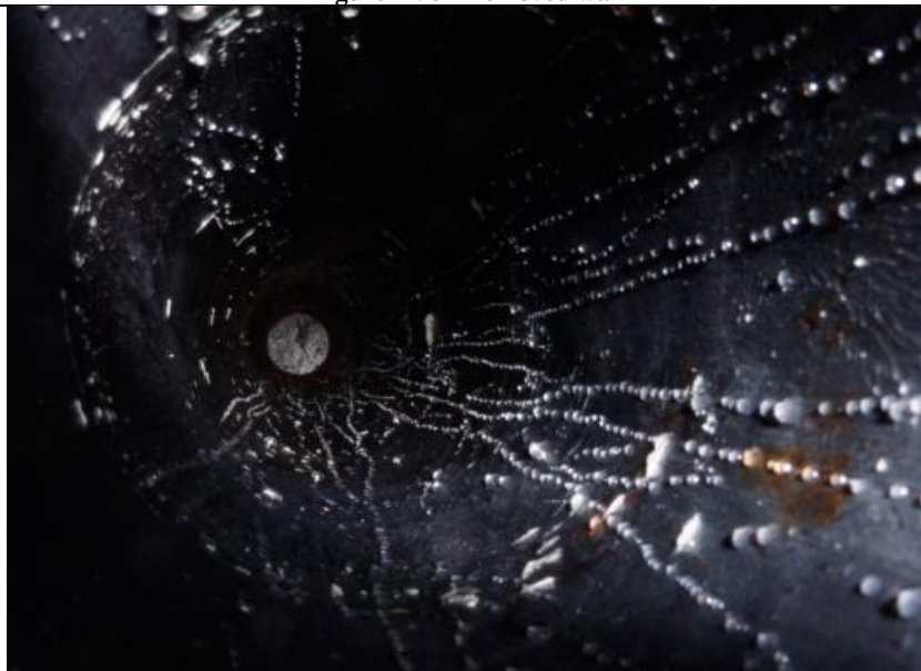
Figure 4-59 - Pipe after wax removal (looking downstream)
