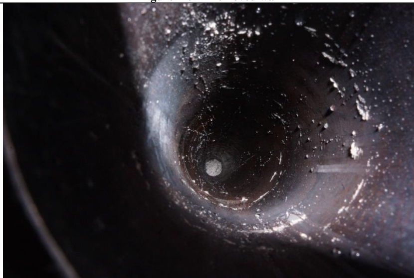
Figure 4-63 - Pipe after wax removal (looking downstream)
