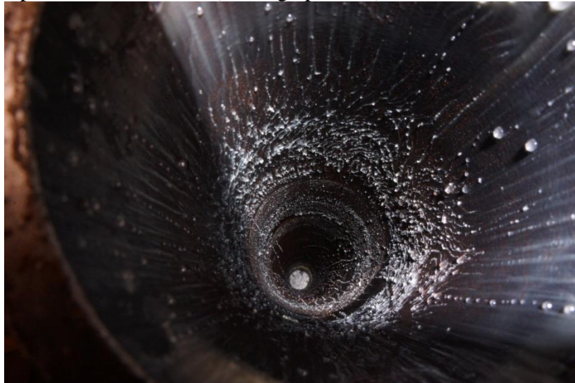
Pipe after wax removal (looking upstream):
