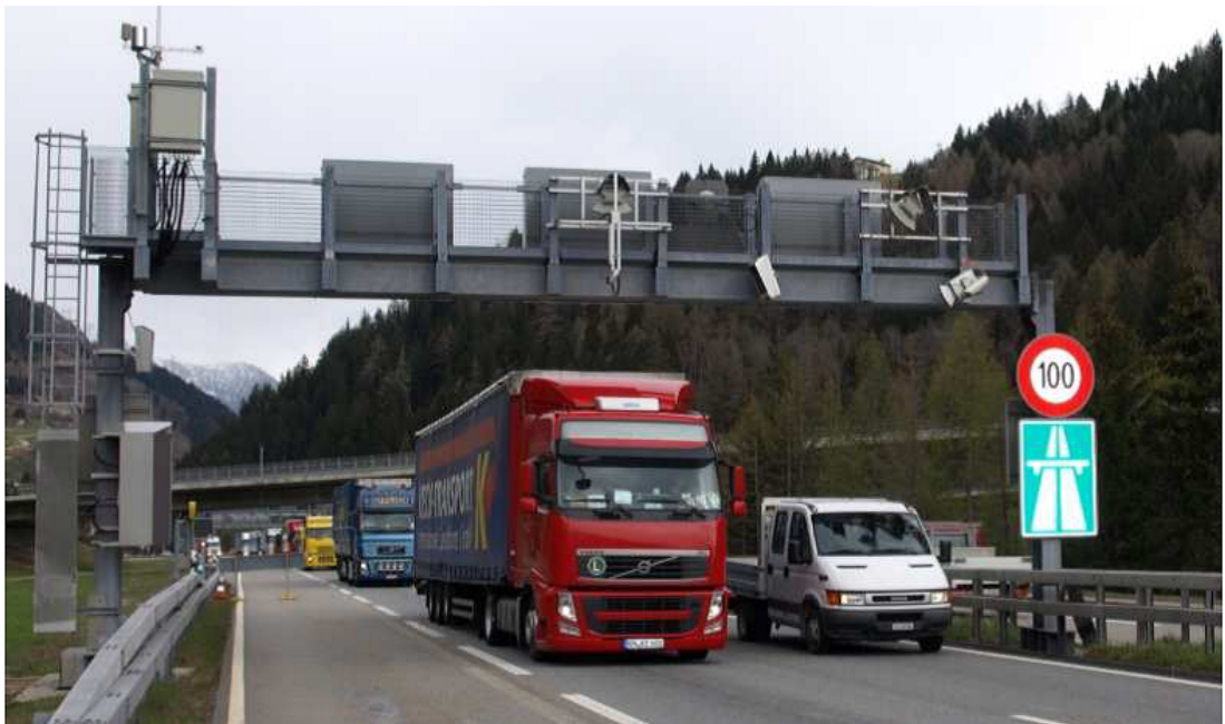
Figure 2.4: Thermal portal at St. Gotthard in Switzerland
