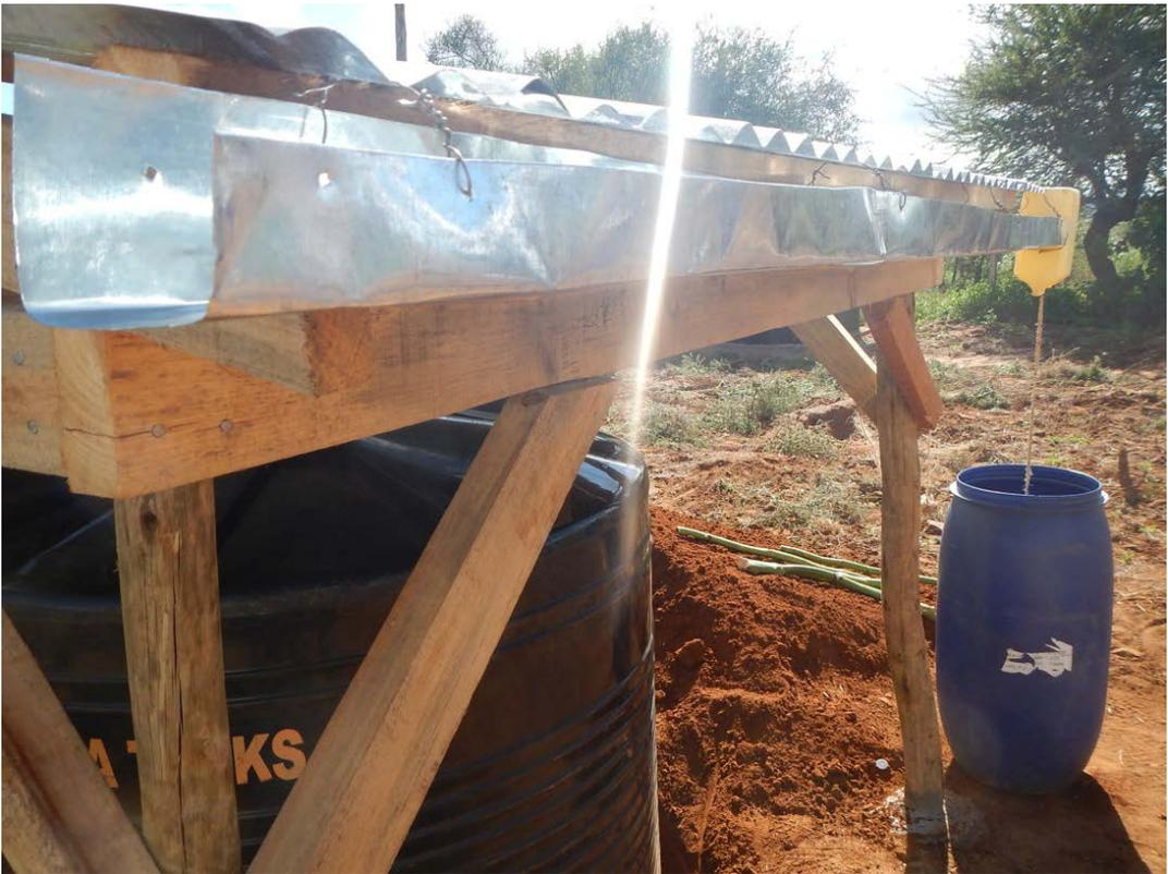
Figure 47 Rainwater harvesting test unit
