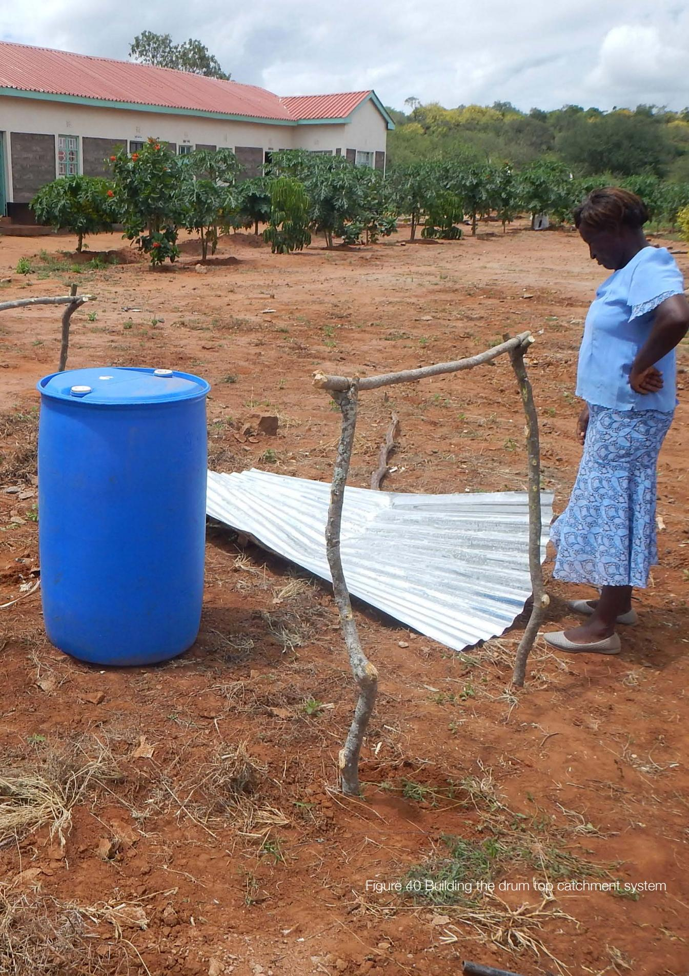
Figure 40 Building the drum top catchment system
