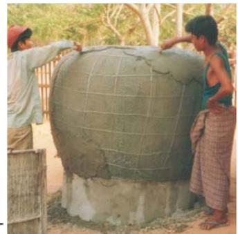
As with the ferro-cement tank there is the need for skilled labor, however the water pots are made smaller than the tanks and may be constructed elsewhere and transported. It is relatively cheap in materials and is relatively quick to construct.
