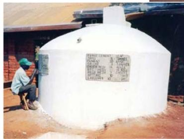
Much like the concrete tank the ferro cement tank is cheap in material and may be produced locally. However, even more skilled labor is needed, and is even more time consuming to construct. Also this type is seen in Ngumbulu, but many have cracked and become useless.
