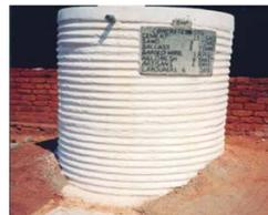
Concrete tanks are relatively cheap in material and must be produced locally, but requires skilled labor and is time consuming. The durability is highly variable and depends on the accuracy in the construction process. In Ngumbulu several of them may be seen, some operational some broken and abandoned.
