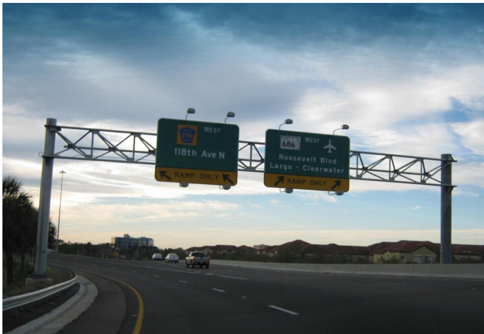
Figure 2-13: Example of a trussed frame Gantry 1 - In Interstate275florida
