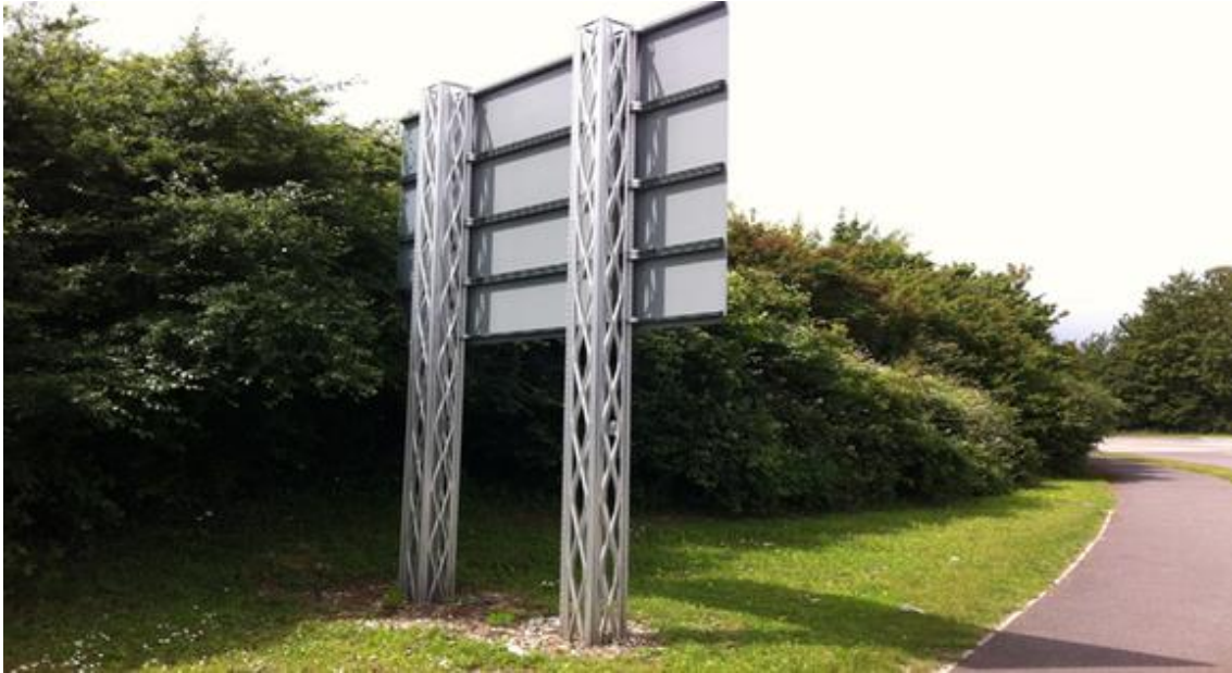
Figure 2-4: Example of a Mast - In Signway
