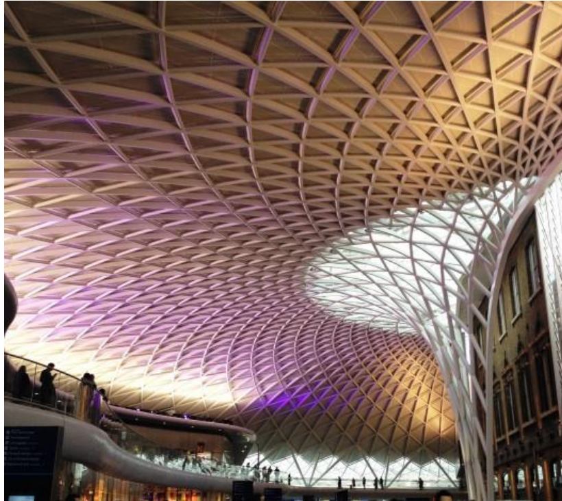
Figure 2-10: Example of a space truss (King's Cross Station, London) – In Now-here-this.timeout.
