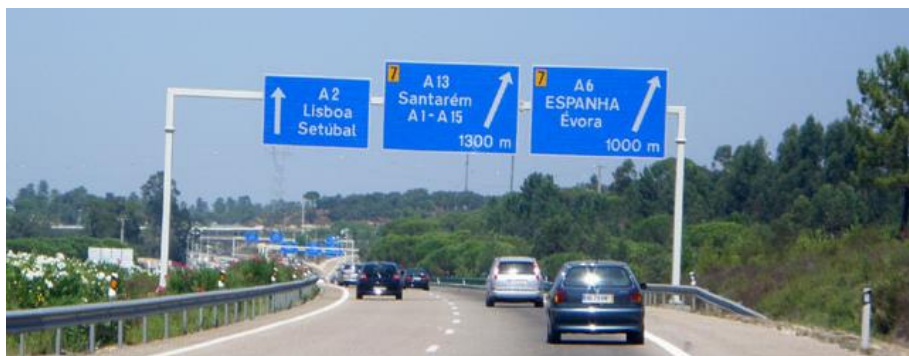
Figure 2-7: Example of a framed Gantry 1 - In Skyscrapercity
