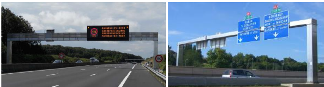
Figure 4-16: Model W : a) with walkway; b) without walkway
