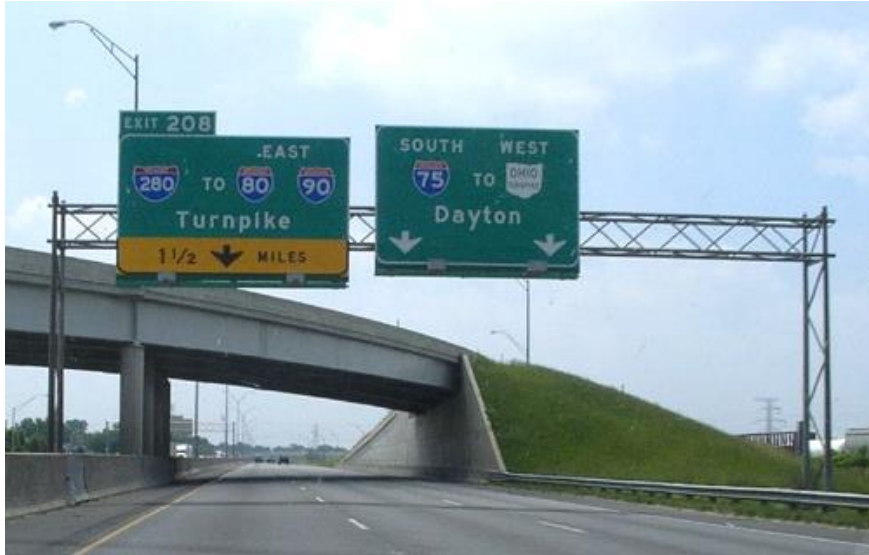
Figure 2-12: Example of a Trussed Gantry 2 – In State-Ends
