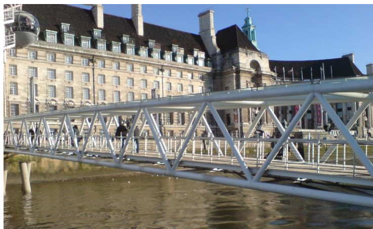
Figure 2-9: Example of a trussed bridge (London) – In Bristol
