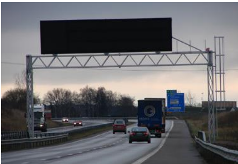
Figure 2-11: Example of a Trussed Gantry 1 – In Sapagroup
