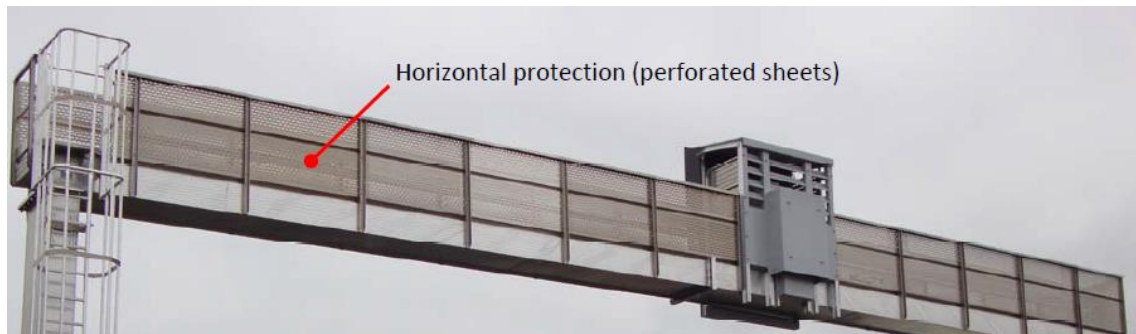
Figure 4-17: Model W: Walkaway's vertical profiles and side perforated sheets
