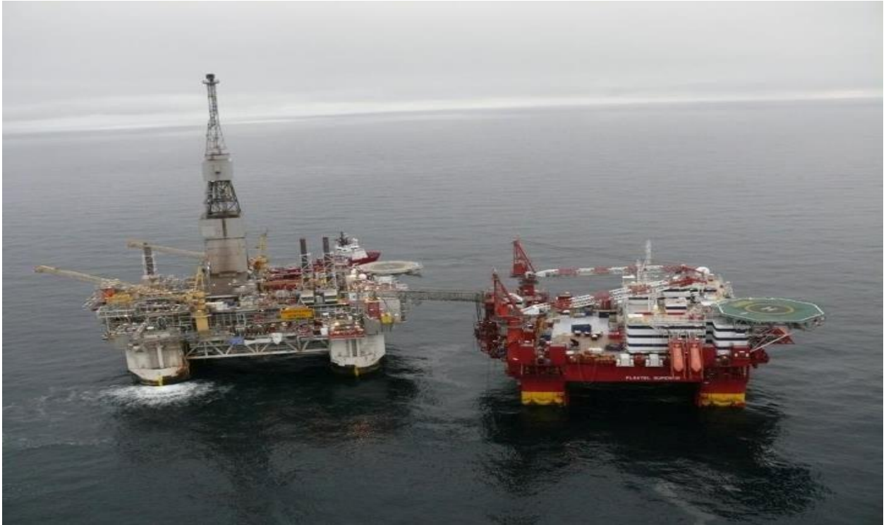
Figure 1.2. Oil and gas platform [3]
