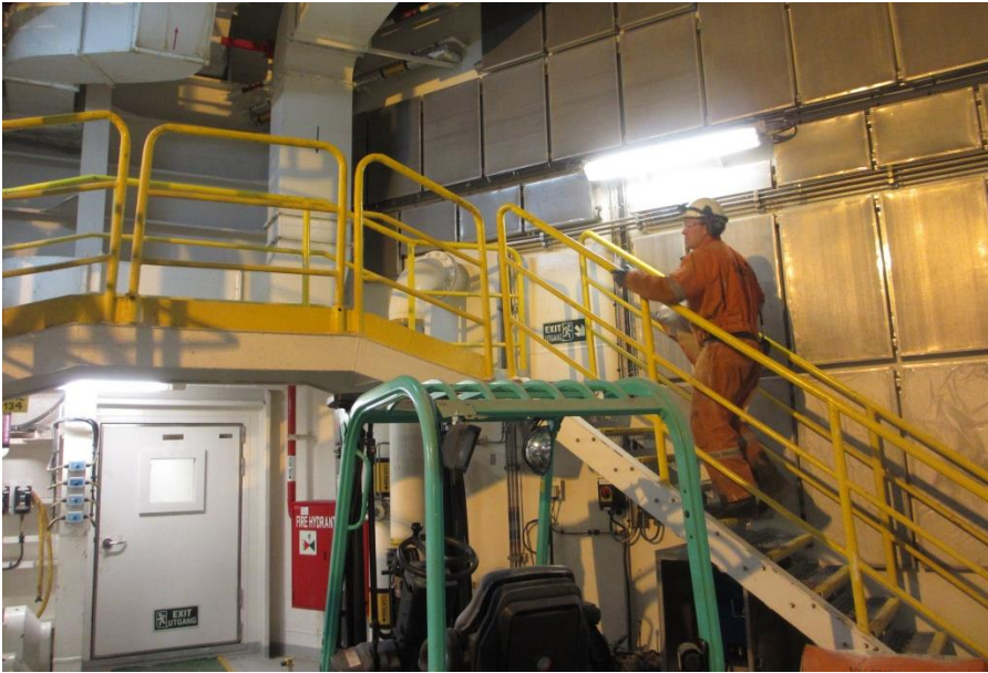
Figure 29 - Stair from sack store to hopper (photo: Sondre Buset Bjelland)
