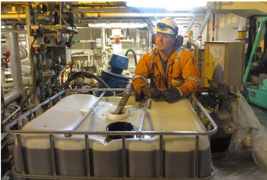
Figure 10 - Adding liquid chemical using the LAS (photo: Sondre Buset Bjelland)
