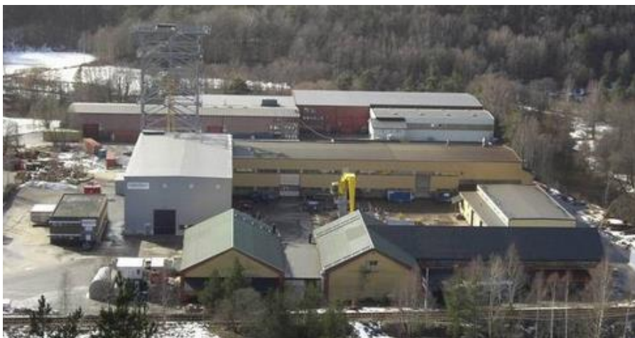
Figure 2 - Test and assembly site in Songdalen, Vest-Agder (courtesy of TTS Group)
