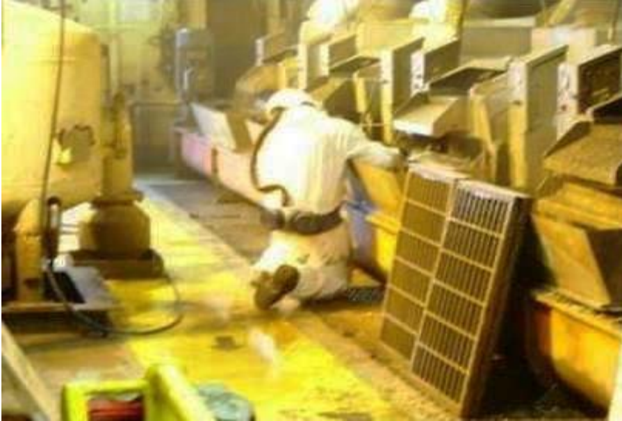
Figure 39 - Before installation of MudCube (source: Cubility)
