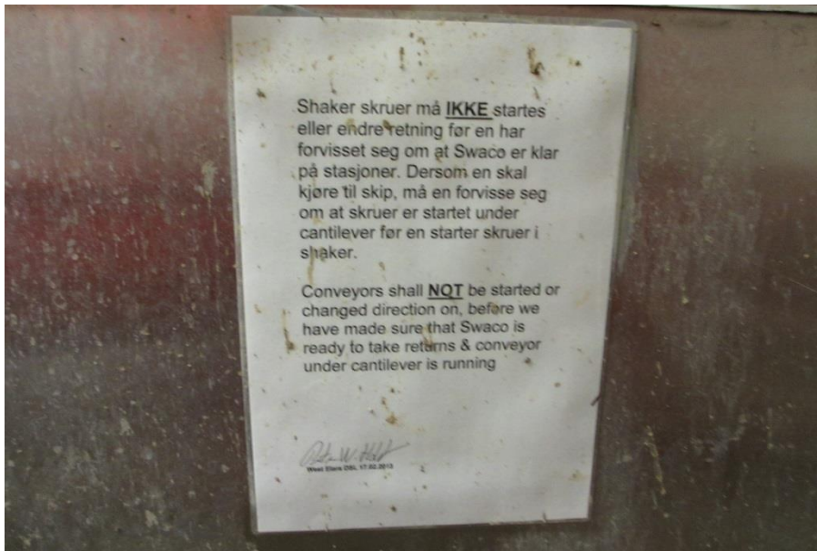
Figure 27 - Warning on screw conveyor control panel (photo: Sondre Buset Bjelland)
