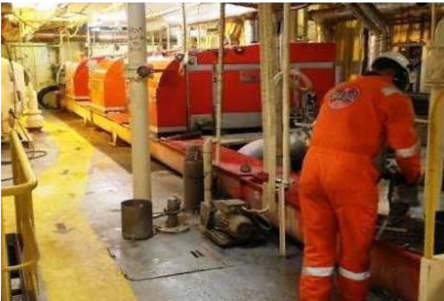
Figure 40 - After installation of MudCubes (source: Cubility)
