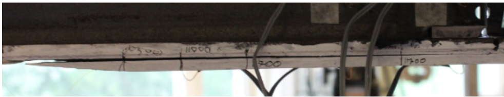
Figure 63: Delamination reaching center of the patch. Beam 33, seen from the back.
