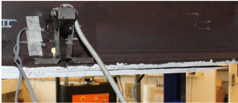
Figure 73: Delamination from the left side. Beam 35, seen from the back.
