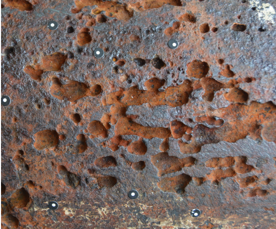
Figure 6.5: Surface conditions of the CLS.
