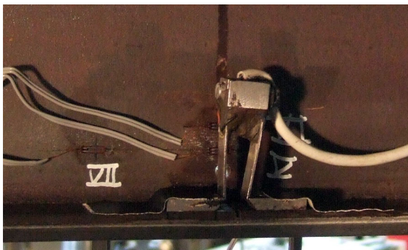
Figure 52: CMOD and strain gauges next to the crack.
