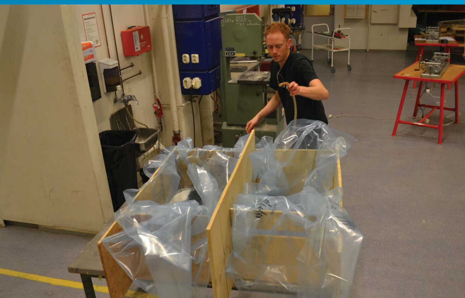
Water reservoir placed over the mold, creating pressure to the carbon fiber in the mold
