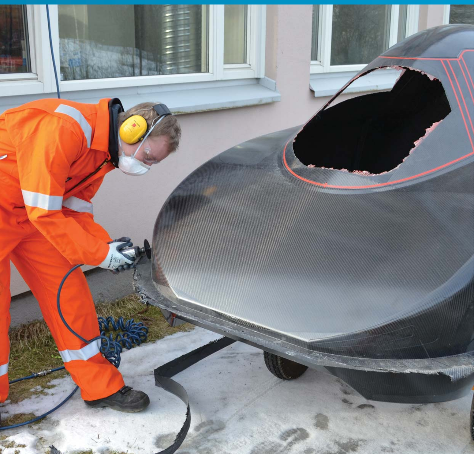
Rough cutting of the monocoque. Thin red tape was used to strengthen the marks from the divider, making sure that the line would not disappear during cutting
