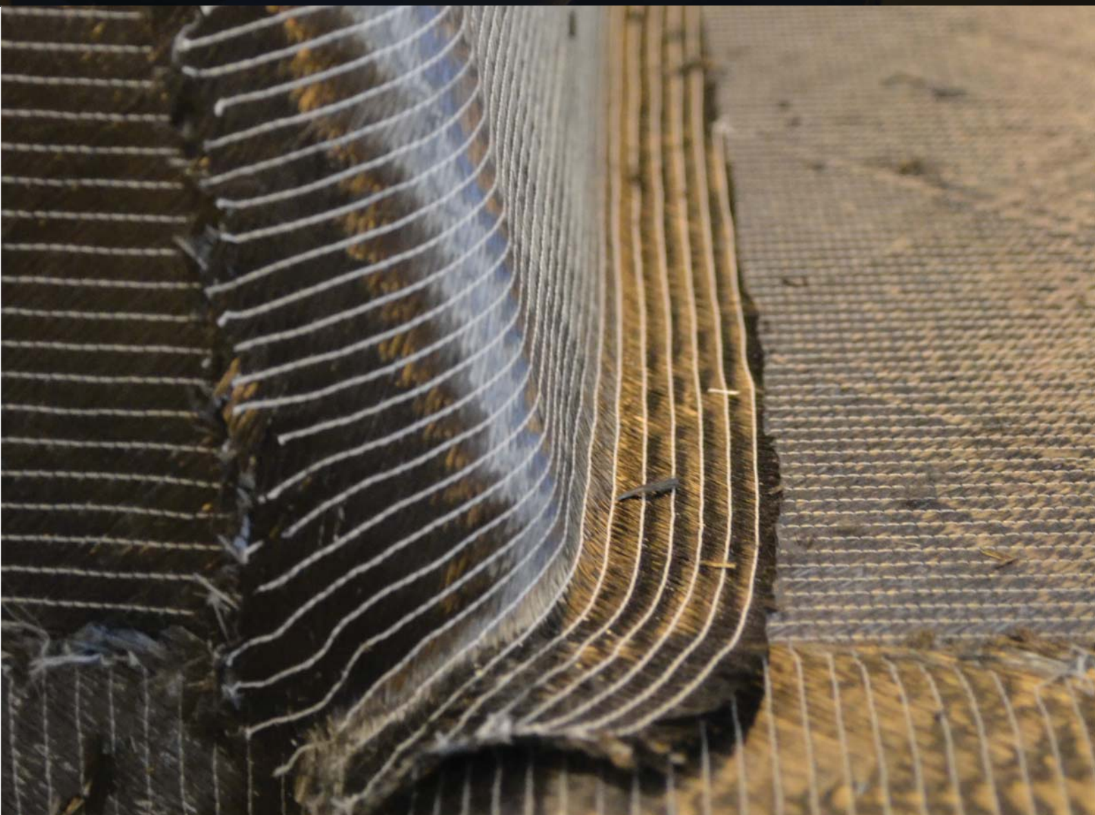
Carbon fiber laid with an overlay of total 40 – 60 mm.
