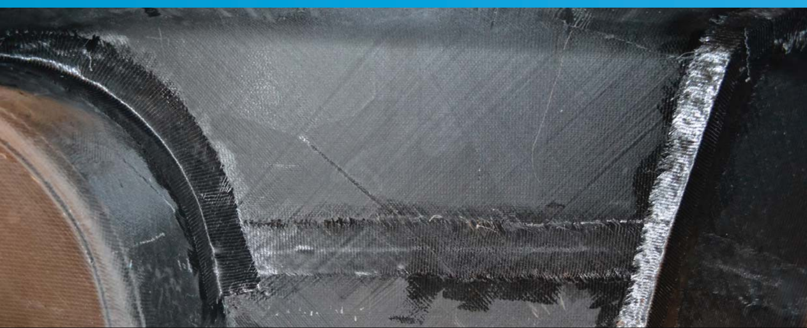
Carbon fiber strips in the seams, holding the three parts together
