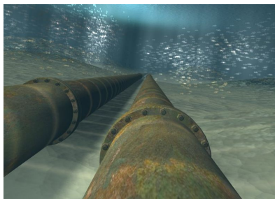
Figure 2.2: A typical pipeline located on the seabed [Subsea World News, 2013b].
