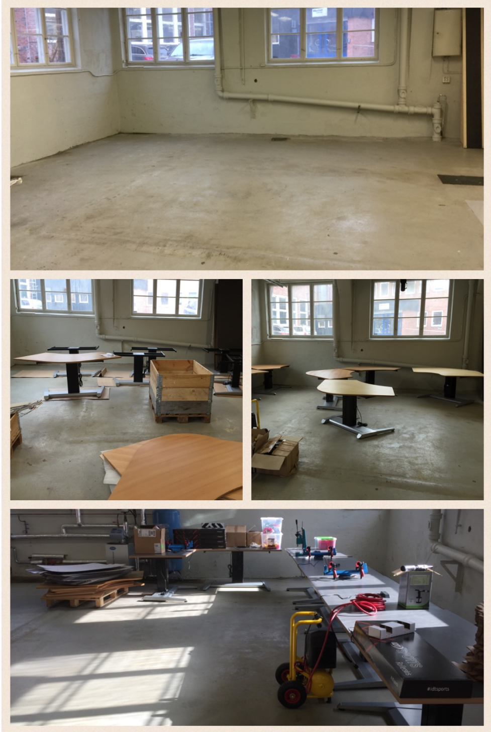
This picture illustrates the building process of NTNU learning factory.
