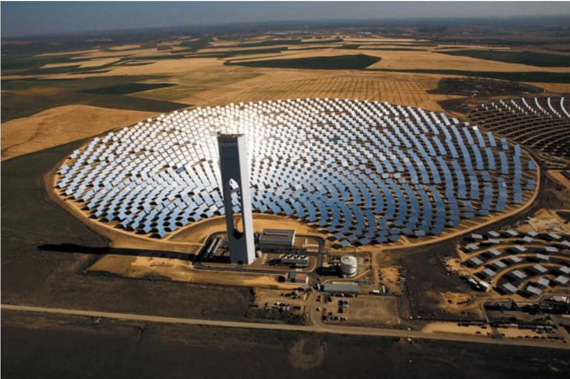
Figure 1: Solar Power Tower plant in Seville, Spain, using solar thermal energy to produce steam for generating electricity in steam turbines [23].
