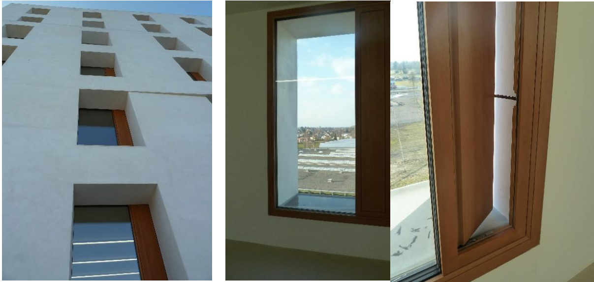
Figure 19 Windows and vents 2226
