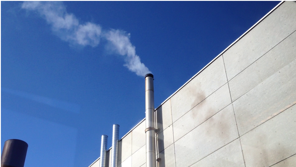
Figure 7.20: White smoke due to retarded start of injection.
