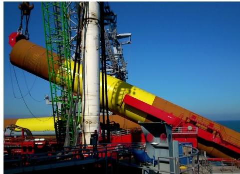
Figure 1.8: Upending on board the installation vessel by 1400 t upending tool (IHC (2016)).
