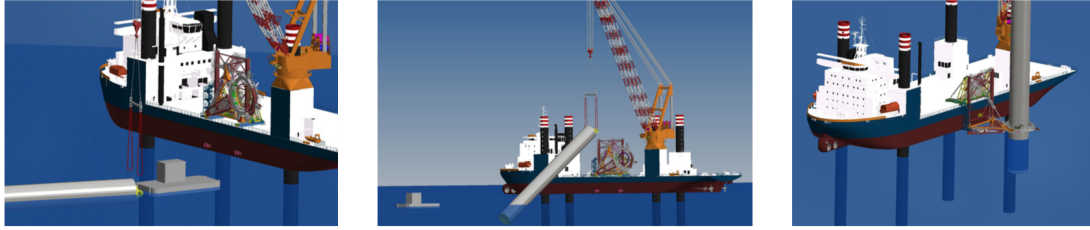
Figure 1.7: Wet tow, upending in water and positioning of monopile (Vellekoop (2015)).
