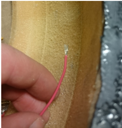
(a) Wire end. The loose individual wires can break off in the terminals.
