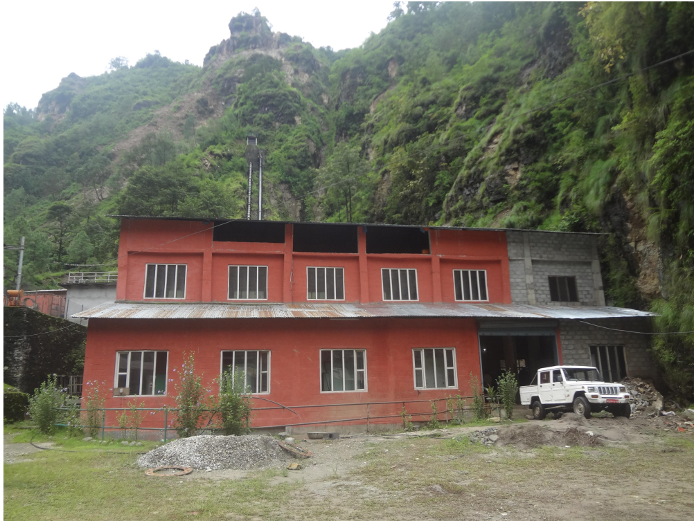
Figure 8.4: Powerhouse of Chaku Khola HPP with penstock in the background.
