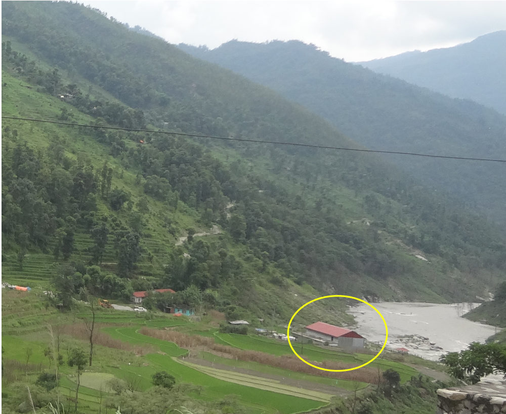
Figure 8.5: Powerhouse of Sunkoshi Small HPP (inside the yellow circle) located on the banks of the Sunkoshi River. It was completely submerged due to the formation of a dammed lake because of Jure rockslide.
