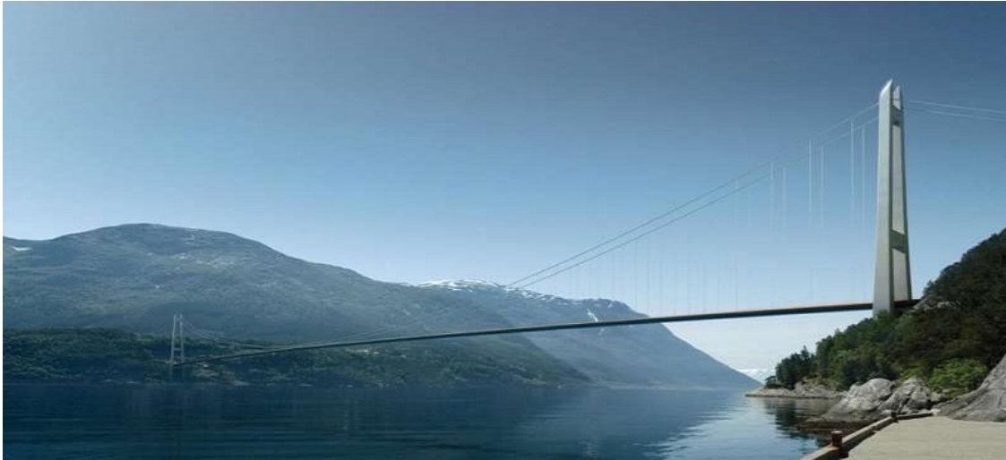
Figure 5.1: Overview of the Hardanger Bridge. The picture is obtained from the websites of the Norwegian Public Roads Administration [40]
