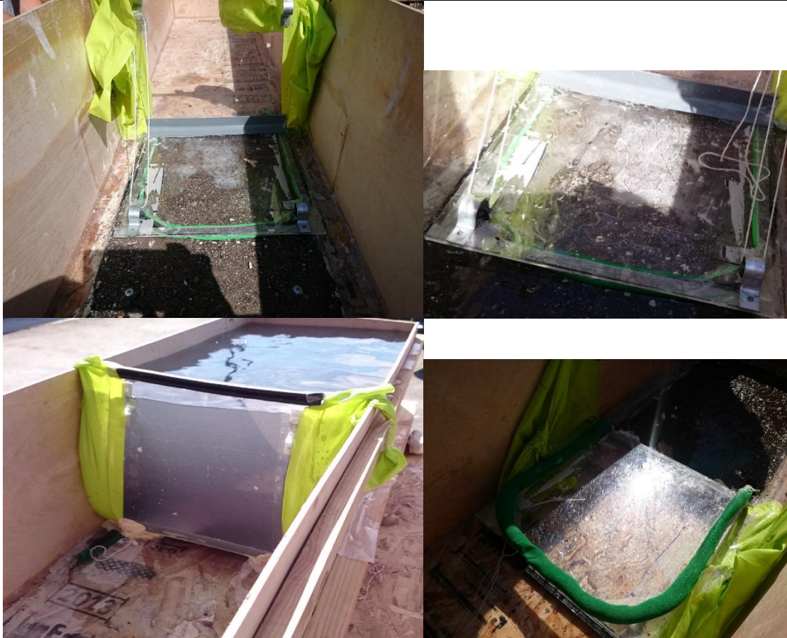
Almost fully sealed at max water height.
