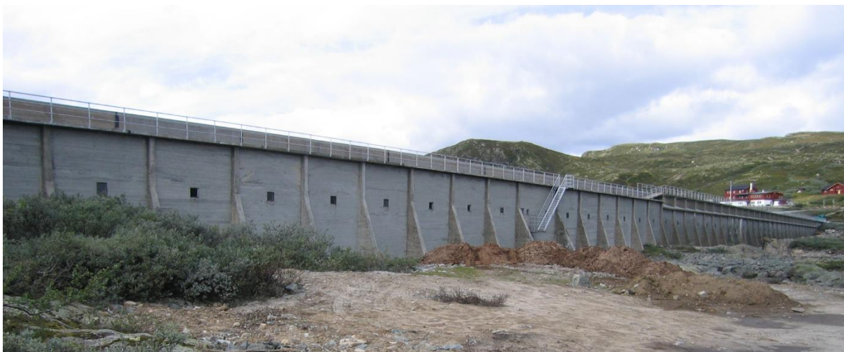
Figure 3.1: Kalhovd dam (Picture: Statkraft)
