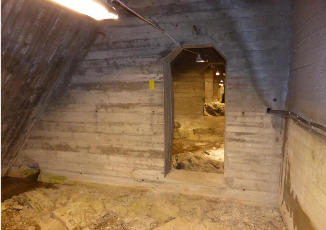
Figure 3.2: Picture of the chosen buttress taken from inside the isolation wall.
