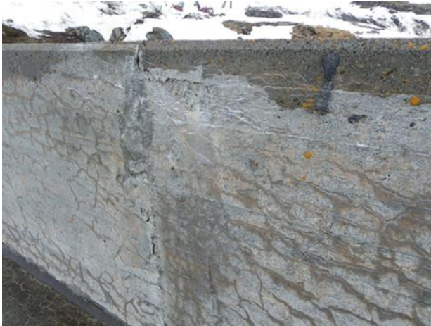
Figure 1.5: The typical map cracking pattern at Votna 1 - May 2015 (Photo: G. Plusquellec)
