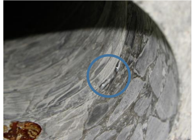
Figure 1.6: Presence of alkali silica gel at Votna 1 - May 2015 (Photo: G. Plusquellec)
